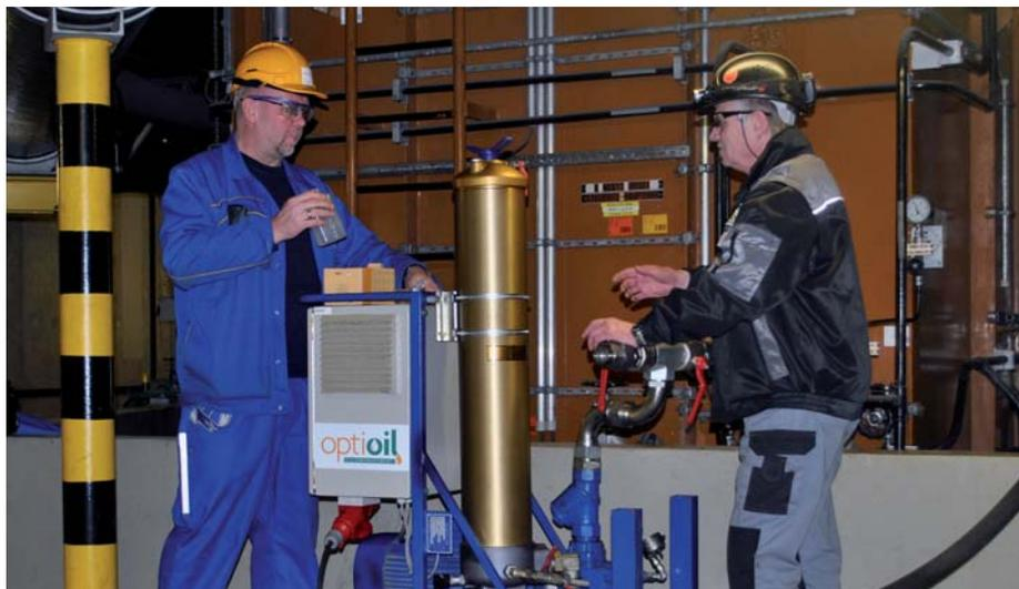
Bypass filtration at a Vattenfall power plant – Maintenance worker and Optioil specialist taking an oil sample.
